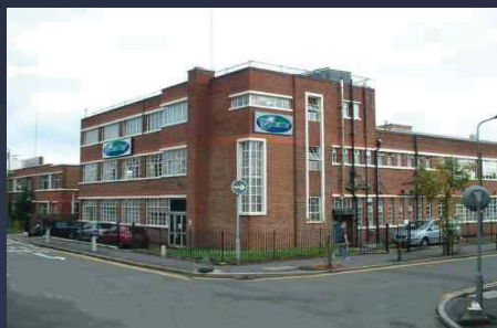
Endecotts head office and production facility in West London
